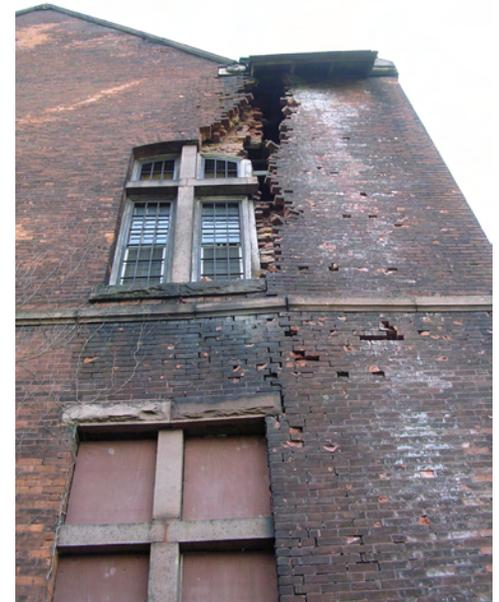
Fig. EX.15 **Brick failure at north elevation in Female Ward I**
