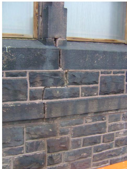
**Fig. EX.14 Step crack through mortar joints in stone facade**
