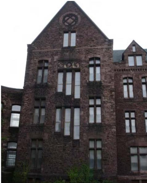
Fig. A.2 South elevation showing decorative features – cornice modillions and brackets, and windows in dormer gable peaks
