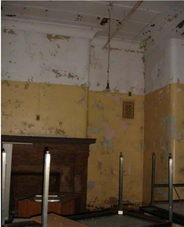
Fig. J.14 **Simpler details - brick fireplace, tin ceilings**
