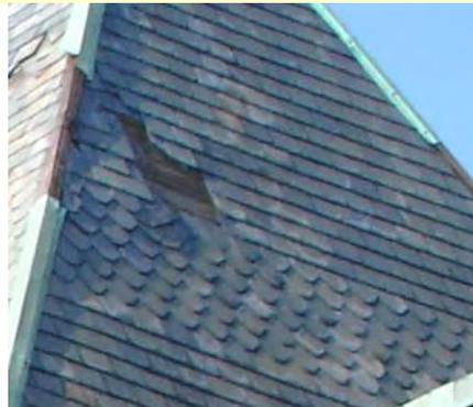
*Slate roof tiles on Female ward I- note rectangular and fish-scale shapes*
