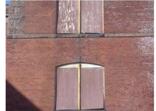
Fig. FDH.3 **Detail of brick jack arch and sandstone beltcourse, keystone, quoins and sill**
