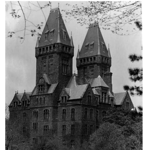
Fig. AB.10 **Historic photo showing original clay tile on tower and slate roof on main building**
