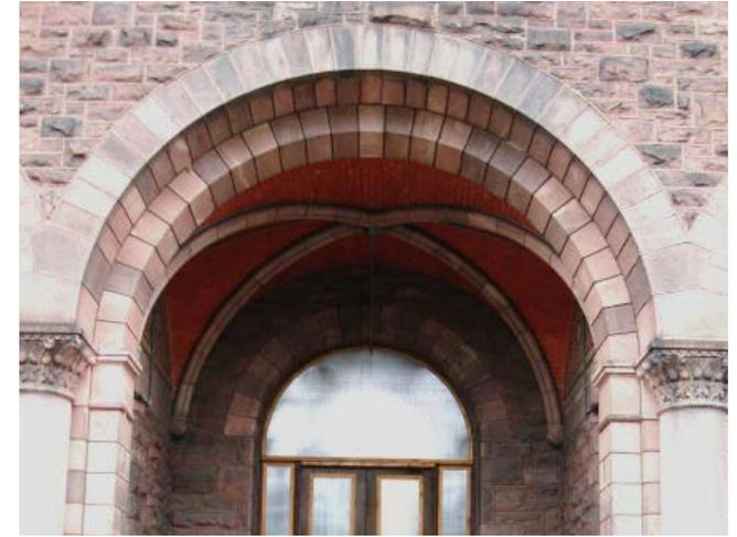
Fig. AB.6 **Brick vaulting at main entrance**
