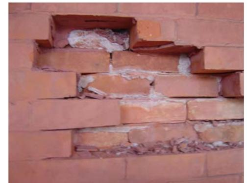
Fig IN.4 Exploratory probe in brick wall
