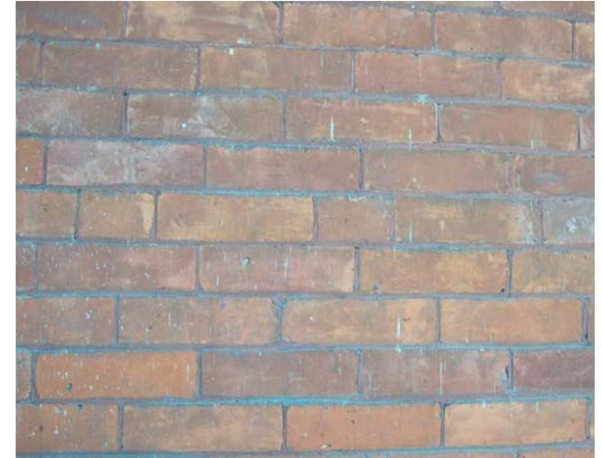
Fig. H.13 Original red mortar evident at porch area
