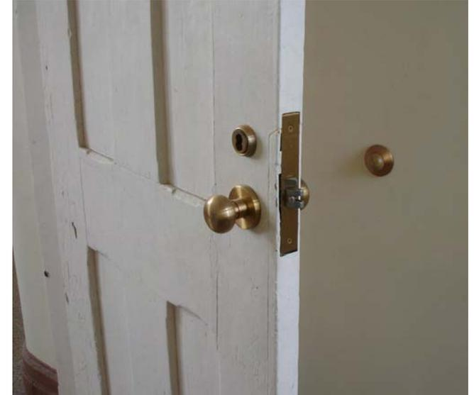
Fig. A.13 Restored door with retrofit hardware
