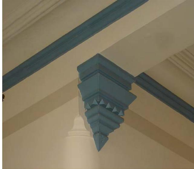
Fig. A.12 Restored plaster molding and bracket
