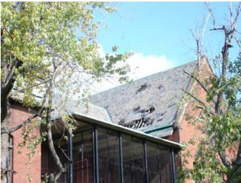
Fig. I.3 **Original slate roof and copper flashings**
