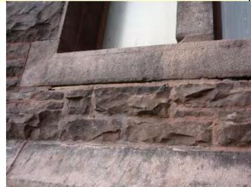
Chiseled, finely hewn sandstone version around openings
