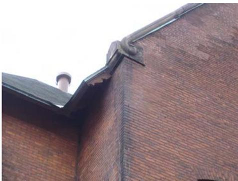
Fig. H.3 **Gable cap stone decorative scroll carving and wooden rafter tail detail**
