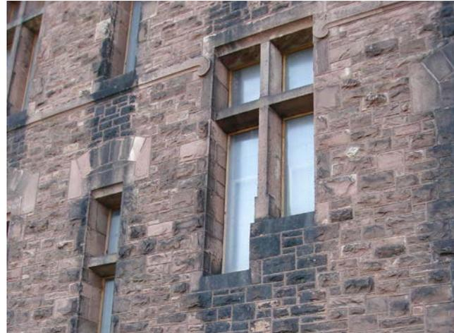
Fig. B.4 Carved scrolled ends where the beltcourse meets the window opening
