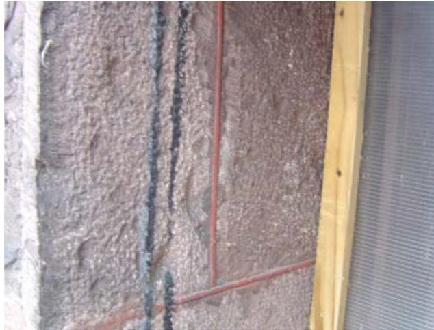
Fig. AB.30 **Original mortar at window jambs**
