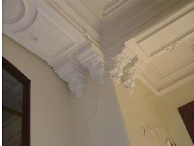
Fig. AB.35 **Decorative plaster brackets and moldings**
